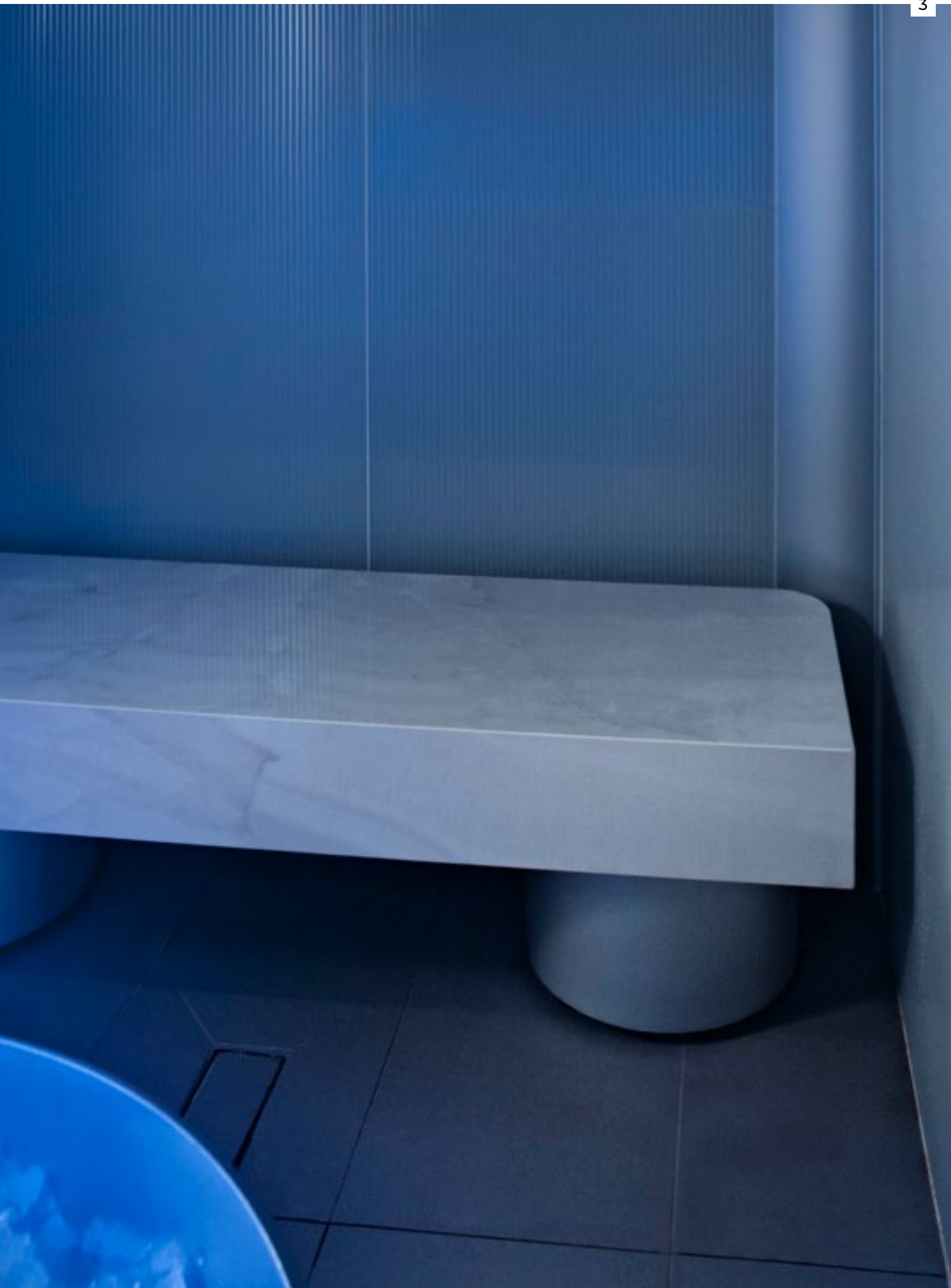
3- The bench is suspended and detached from the wall, making cleaning operations easier.
