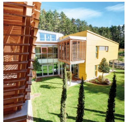
Casa Sebastiano Coredo - Italy
